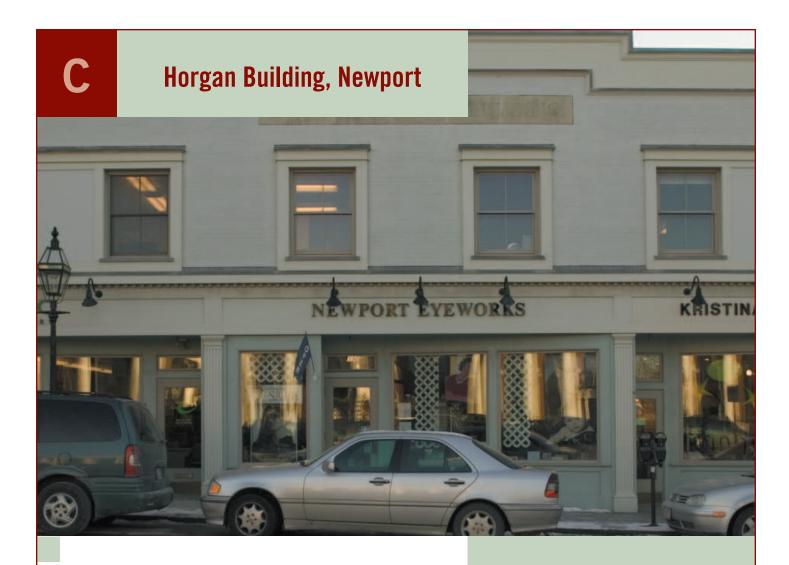
Exterior face lift to the Horgan Building in downtown Newport. All existing glazing was removed and replaced with modern glass. The brick veneer of the building was dressed up with fluted cedar columns and raised panels. The building was capped with lead coated copper.
