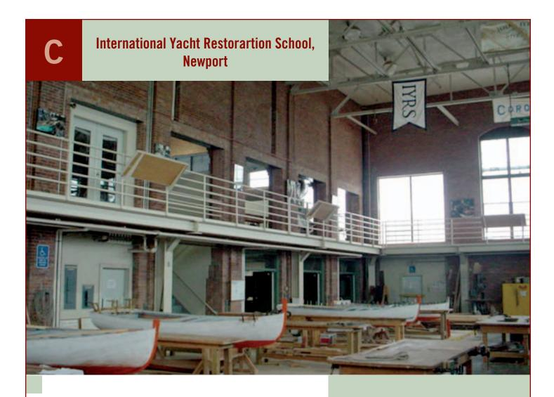
Installation of a second floor, steel framed mezzanine to increase shop space. Installation of a steel catwalk that provides the public with a bird's eye view of the boat restoration projects being carried out. Local code compliance.
